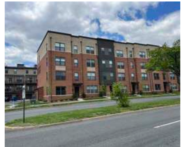
12 Metro Square Condo Complex
