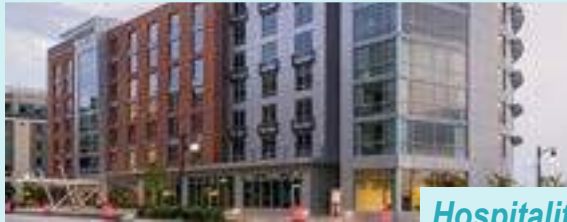
Limited-Service Hotel Hyatt Place National Harbor (Oxon Hill, MD)
