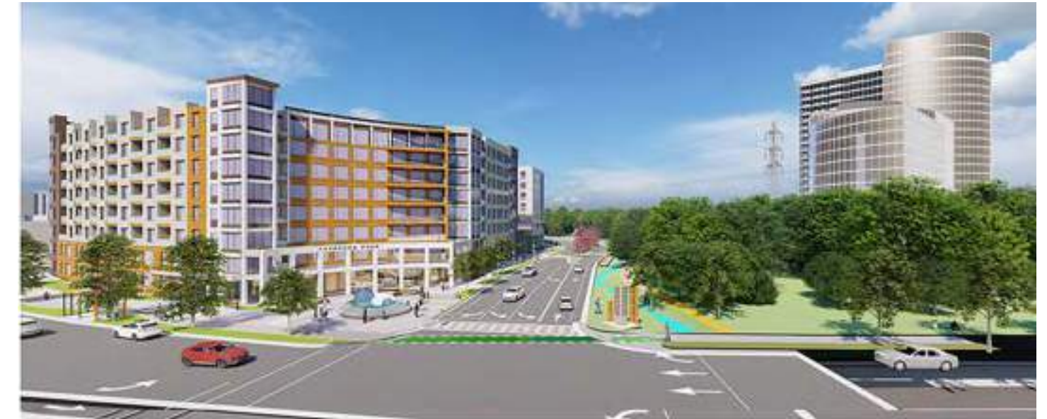
View 1 one of the Fairbrook development options: 8-story residential, new Fairbrook Dr, Sugarland Bridge Park, and 11- & 19-story office buildings
