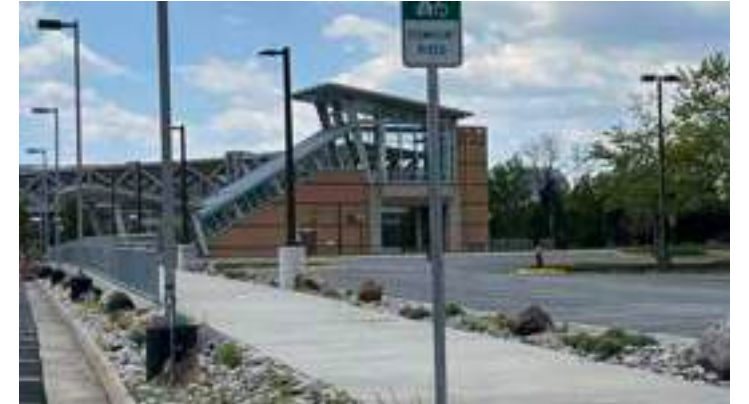
④ Herndon Metro Station, pavilion and path to Herndon Parkway
