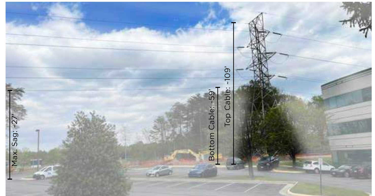
View of transmission Tower A (see exhibit on opposite page)
